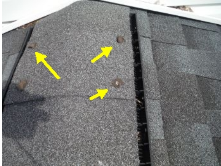
Exposed fasteners
