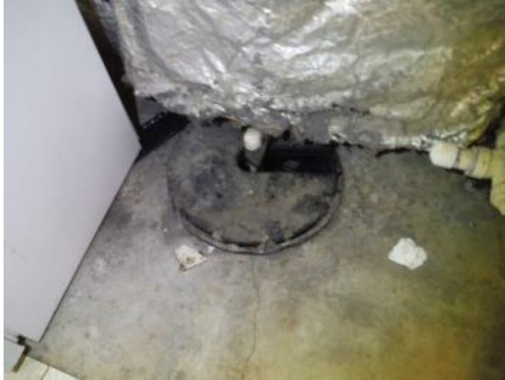
Missing sealant.
