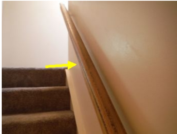
Handrail loose
