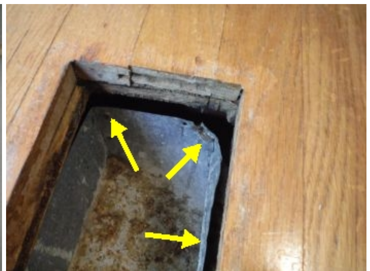
Missing sealant
