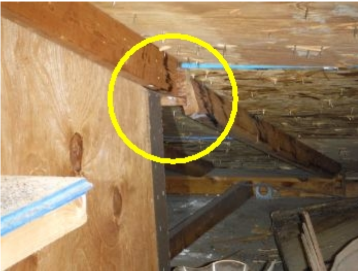
Improper attachment
