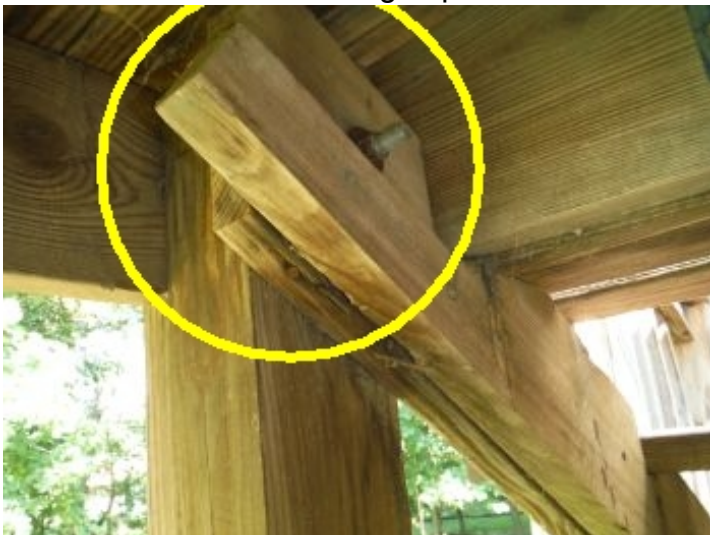
Improper connection.
