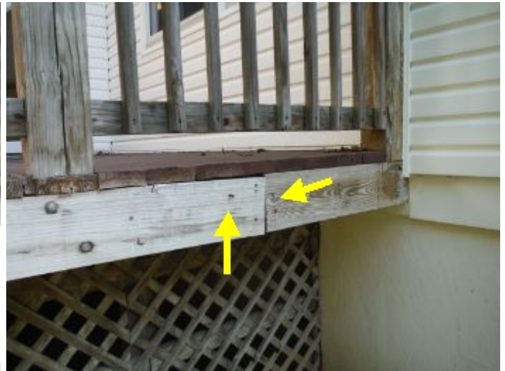
Loose fasteners
