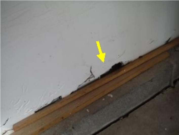
Seal all gaps/openings.
