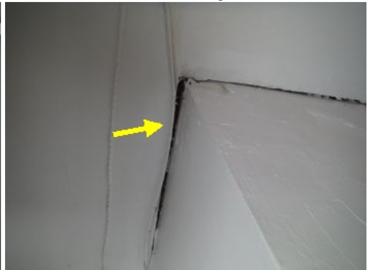
Seal all gaps/openings.
