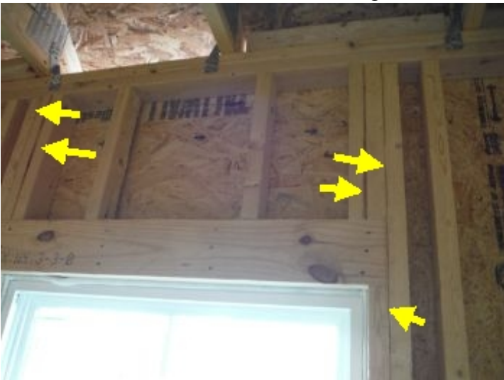
Missing sealant
