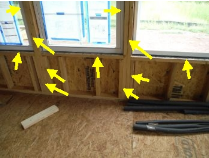
Missing sealant
