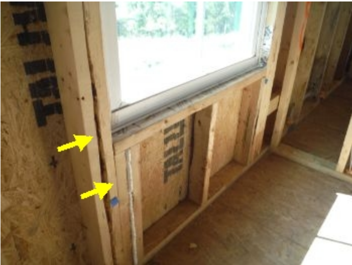
Missing sealant
