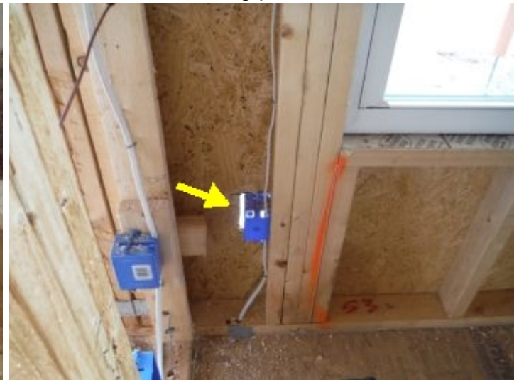
Missing sealant
