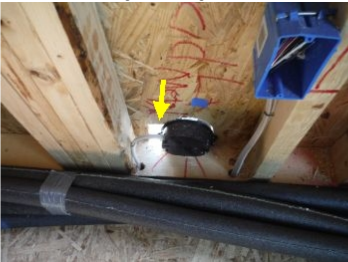
Missing sealant
