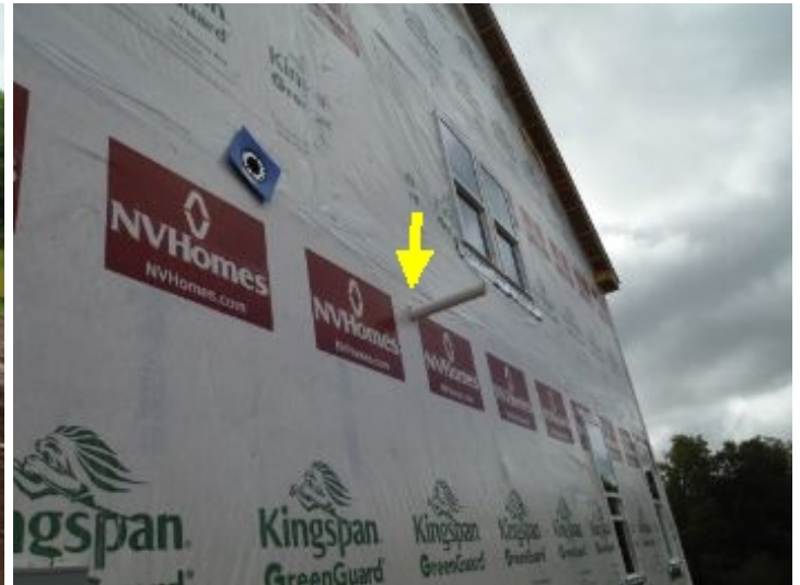
Flashing Missing
