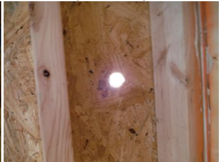
Damaged sheathing
