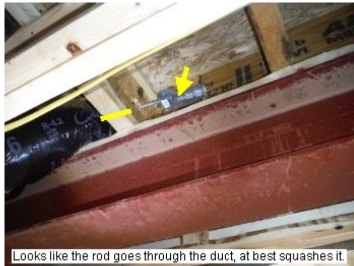
Missing fastener
