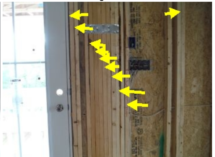
Missing sealant
