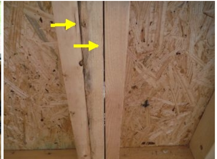
Missing sealant Study
