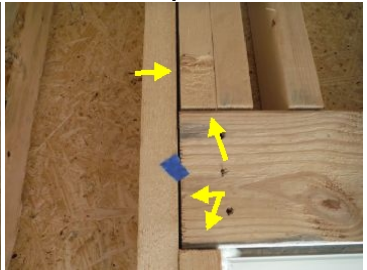
Missing sealant
