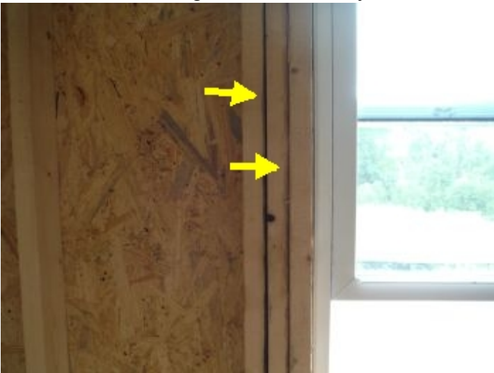
Missing sealant
