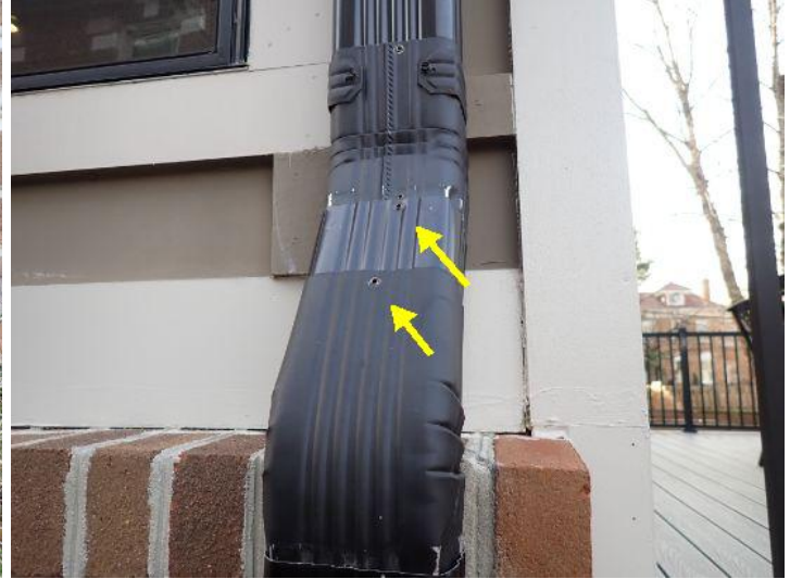
Missing fasteners
