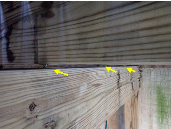
Missing bearing
