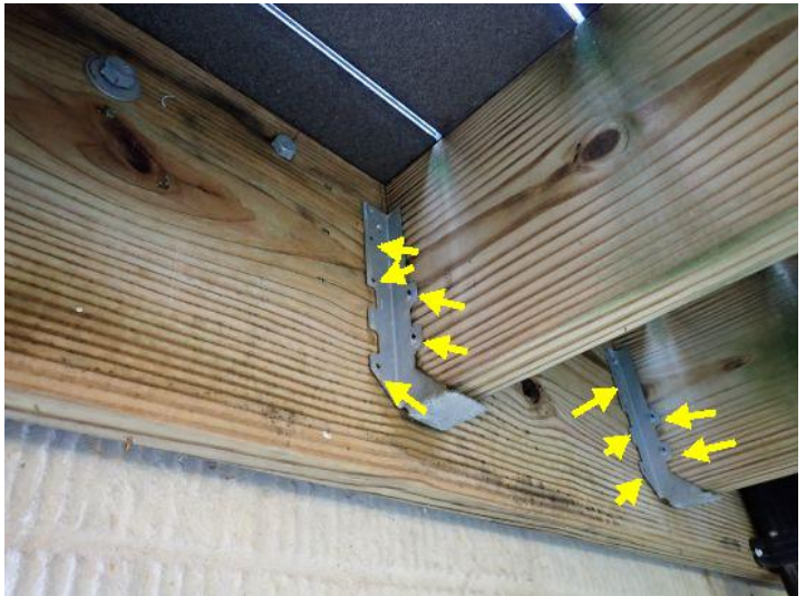
Missing fasteners
