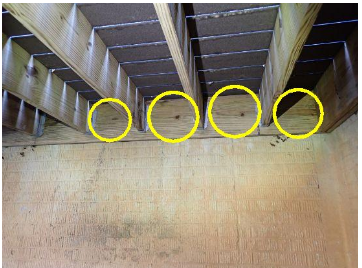
Missing fasteners
