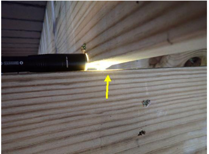
Missing bearing
