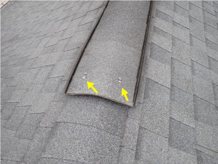
Exposed fasteners
