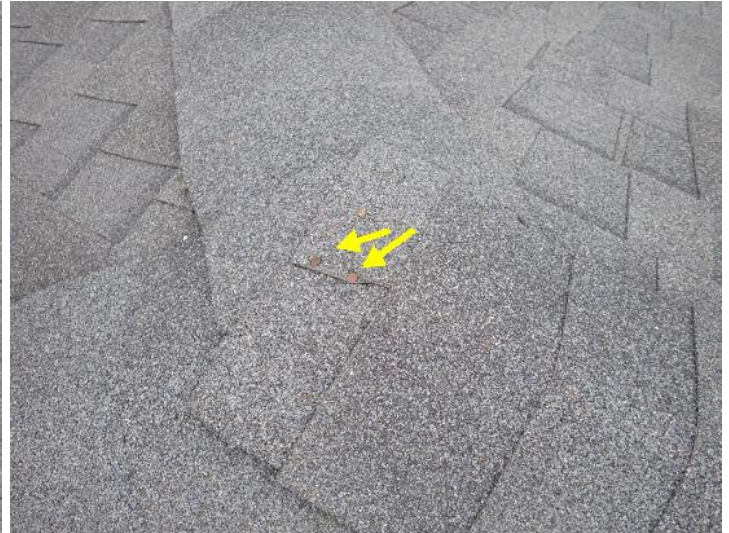
Exposed fasteners
