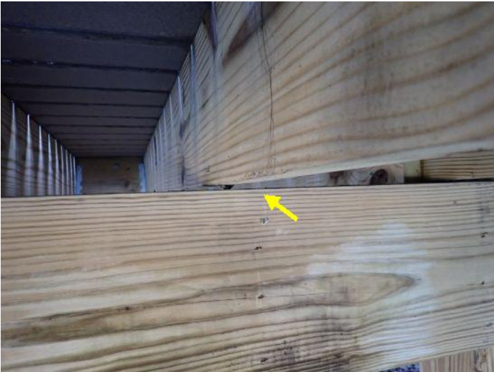
Missing bearing
