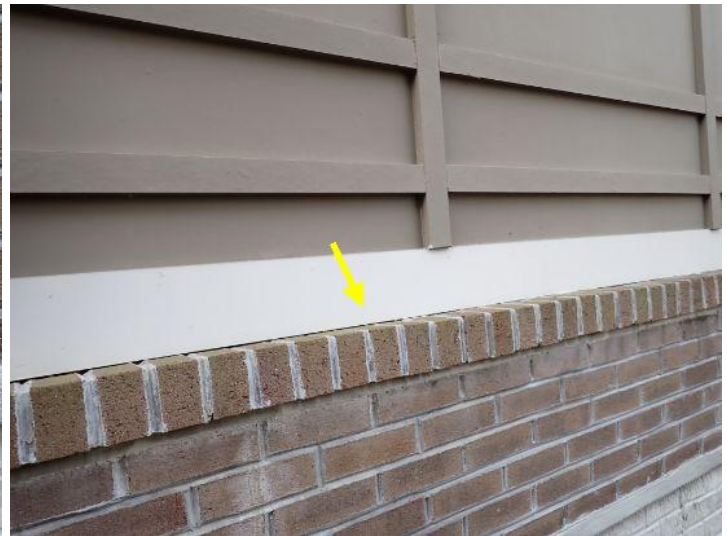
Missing flashing
