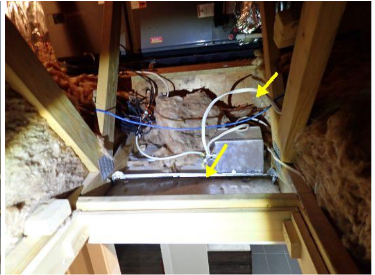
Low or Missing insulation
