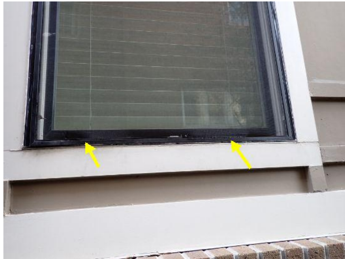
Damaged Screen
