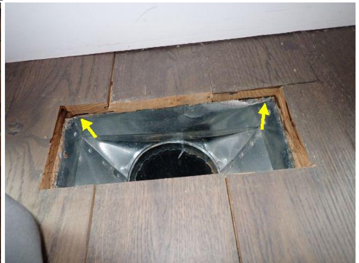
Missing sealant
